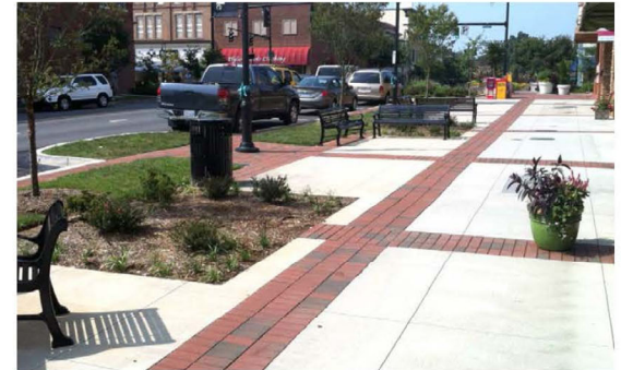
BRICK AND CONCRETE COMBINATION SIDEWALK
